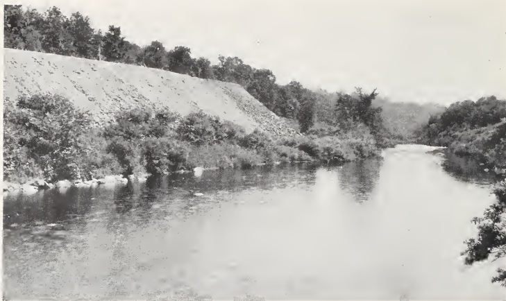
a. View looking down the Shepaug River from below the site of the proposed dam. Part of the dump from the tunnel excavation is shown at the left.
