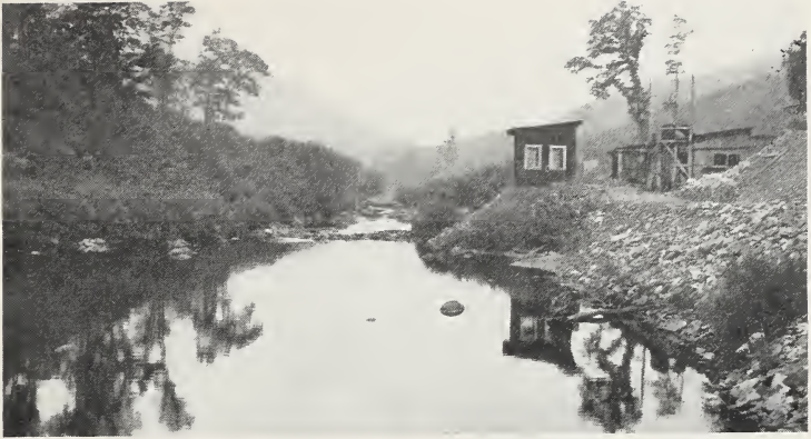
a. View looking up the Shepaug River Valley, soon to be turned into a reservoir. Tunnel entrance to the right of the shacks. Photograph by B. H. Walden.
