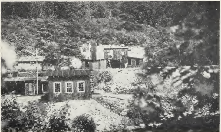
b. View looking into entrance of tunnel from across the Shepaug River, along the line of the proposed dam.
