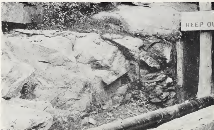
b. View showing the massive character of the Brookfield diorite at the entrance to the tunnel east of the Bantam River crossing.
